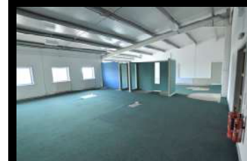
First floor mezzanine
