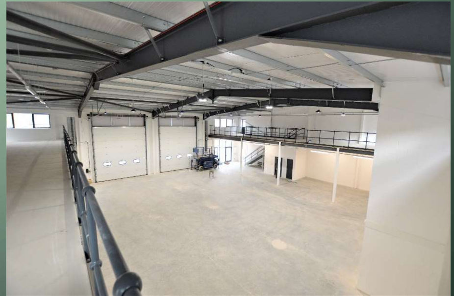
Under floor heating with air source heat pumps, intelligent LED lighting, mezzanine, shower and toilets
