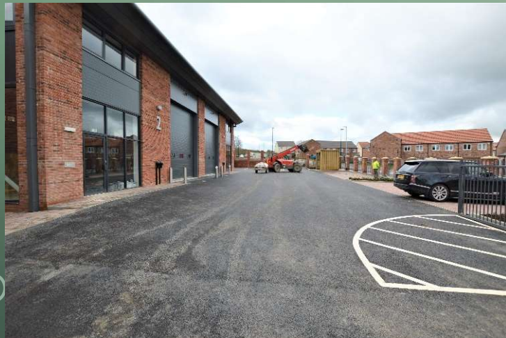
Anti-ram bollards and 2 electric chargers per unit
