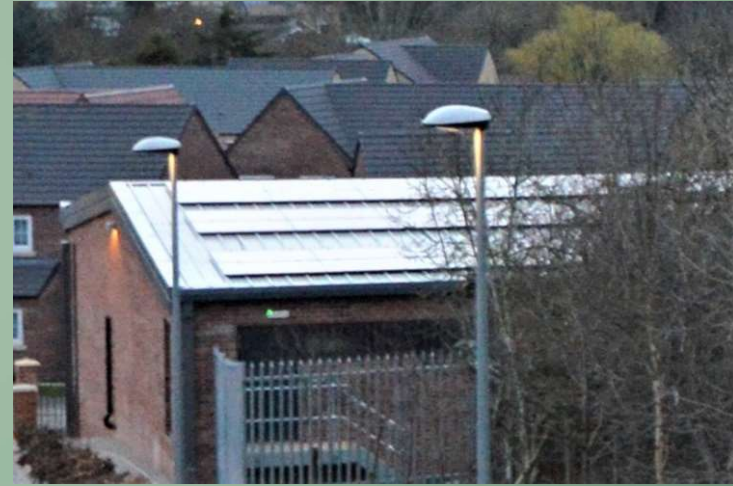
Solar panels generate electricity and powers heating
