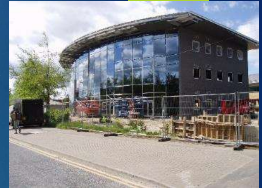
Facilities at Hornbeam Park
